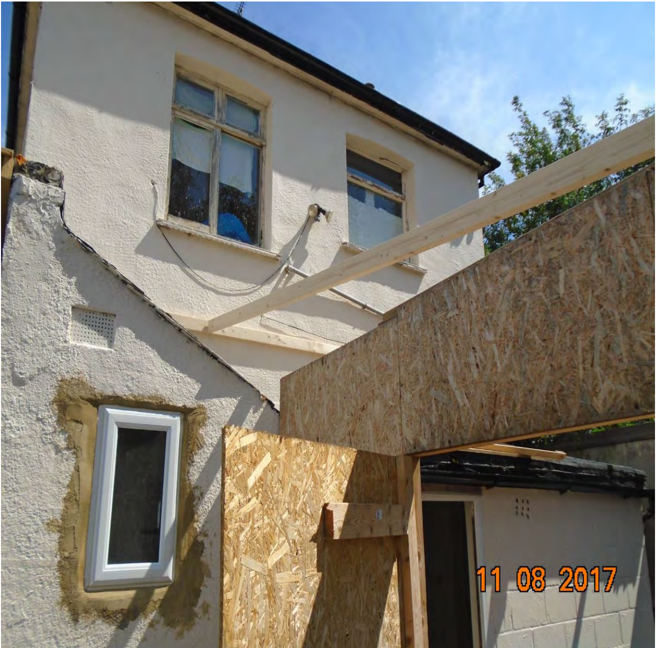
Wall plate and joist at rear of premises
