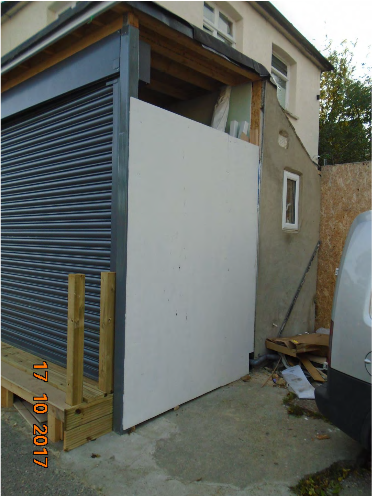
Side Extension viewed from west side
