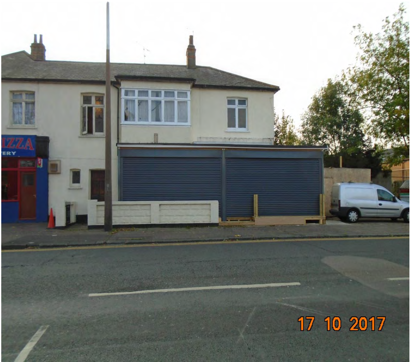
Side Extension viewed from Fairfax Drive
