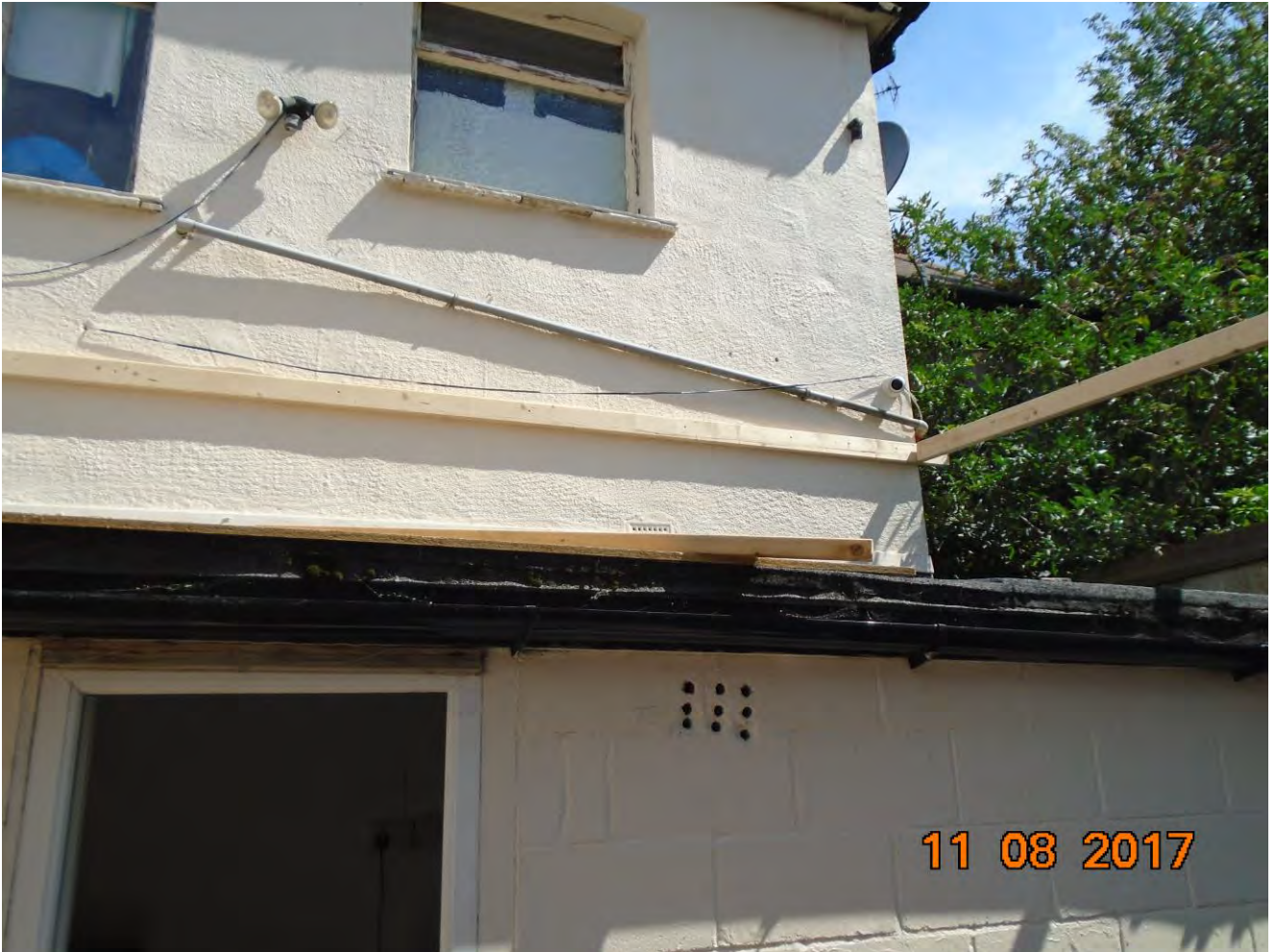
Wall plate and joist at rear of premises
